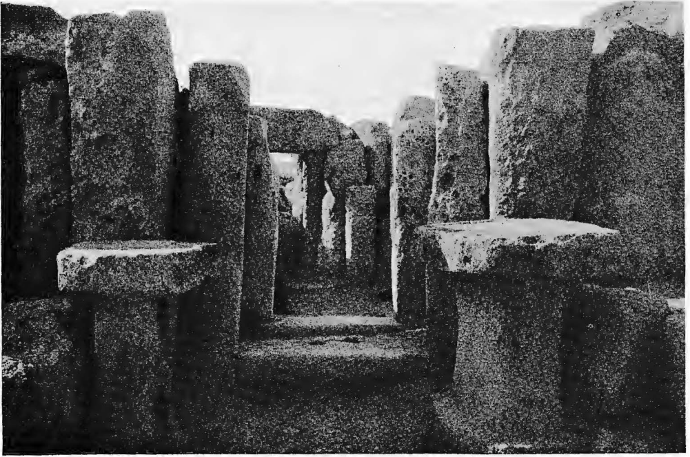
A STONE AGE TEMPLE SHOWING SACRIFICIAL TABLES IN THE FOREGROUND: MALTA
